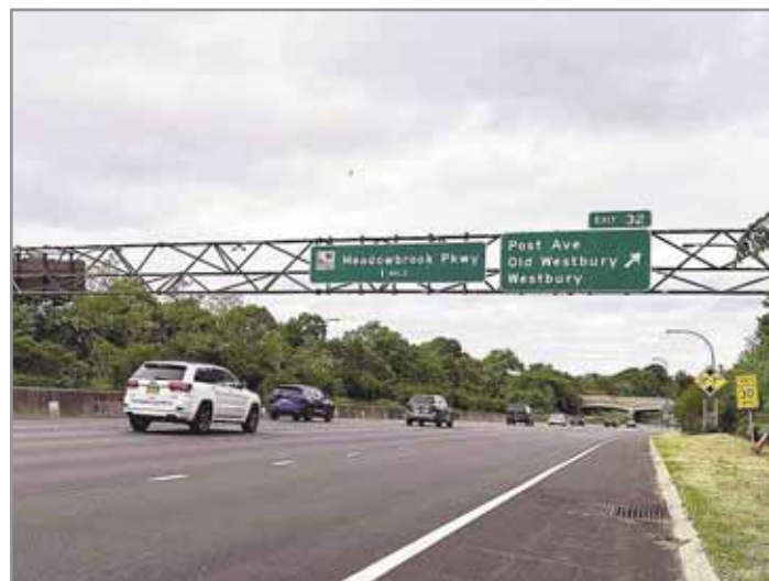
Newly repaved westbound Northern State Parkway is seen Sunday.
